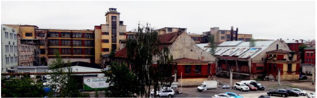
The main knitting, dyeing and bleaching workshops. Friday, July 22, 2016 Photo by S. Gorbatenko
