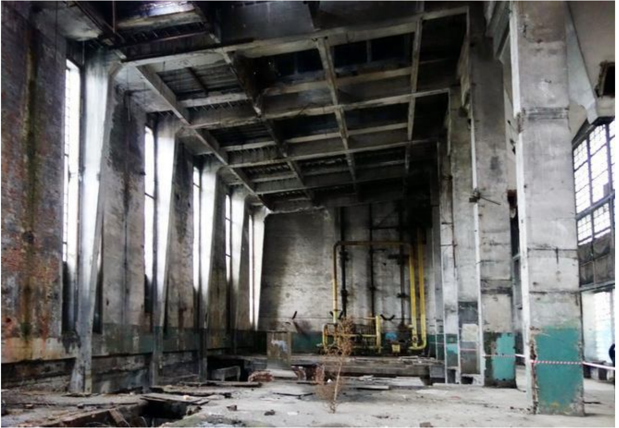
Power station. Boiler room interior. March 17, 2017 Photo by N. Dushkina
