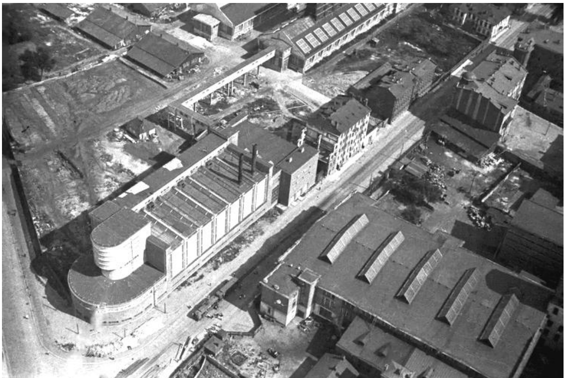
The Red Banner Factory under construction. Aerial photo. 1920s
