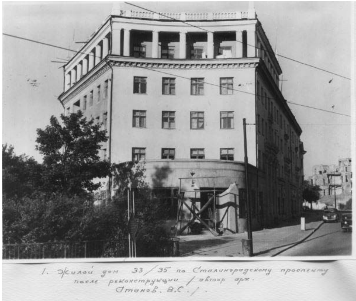
Picture 4. Apartment house #33/35 on Stalingradsky avenue (now #33-37 Mira avenue) after reconstruction [2]
