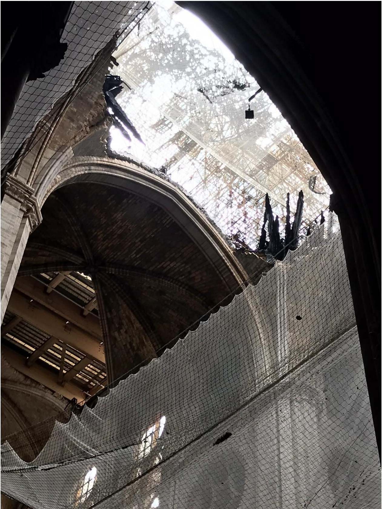
The crossing of nave and transept as it looks today
