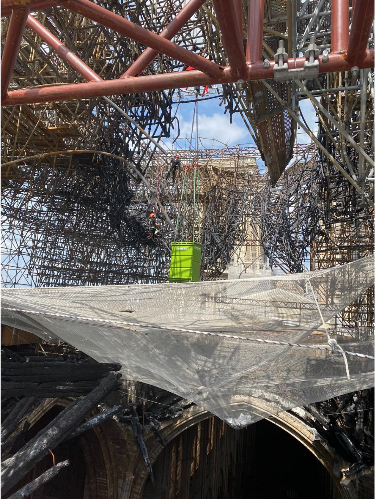
Roped-up workmen dismantling the fused scaffolding
